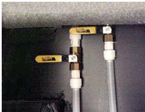
Water Line Drain Valves in Water Center Models 34SH & 36SG
