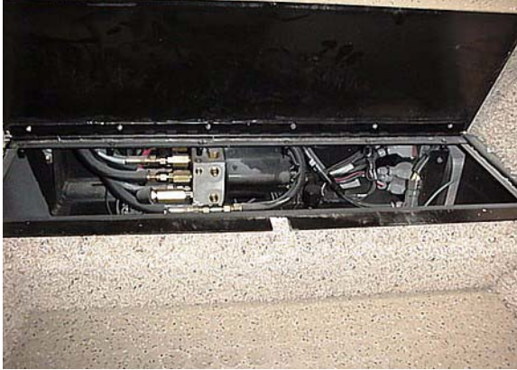
Hydraulic Pump beneath Entry Step
