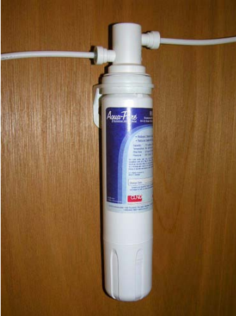
Water Filter Assembly (Located below Galley Sink)
