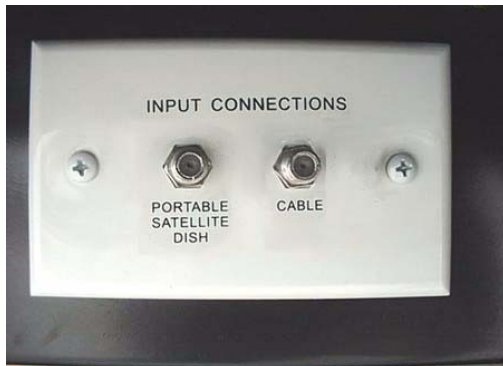
Exterior Connection for Satellite Dishes and Cable TV (In Utility Compartment)
